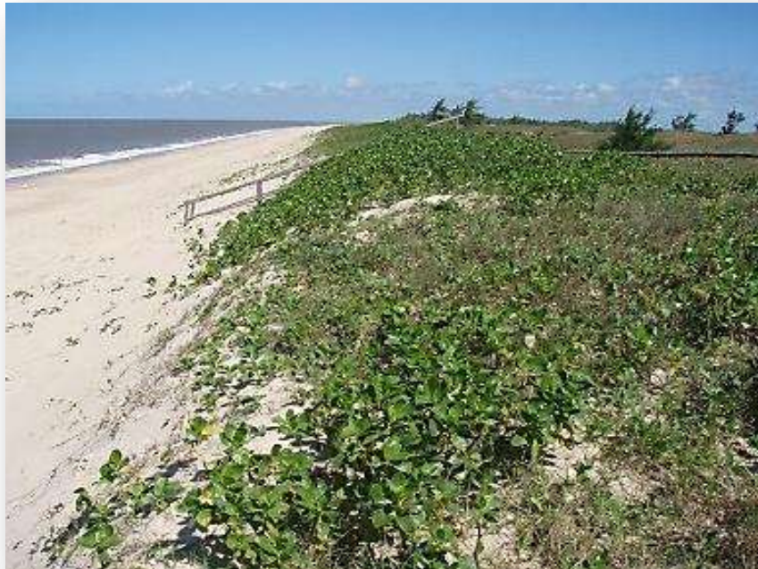
Figure 7.4: Example of a vegetated dune at Beira with sufficient volume and height to protect landwards areas from storm erosion or coastal flooding.
